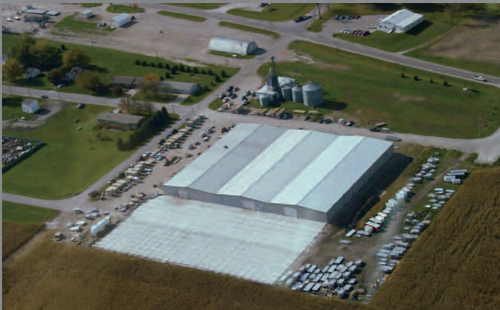
Aerial view of Aluma factory
